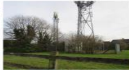
Figure 7: View of telecommunication masts and reservoir north of Parcel B.
